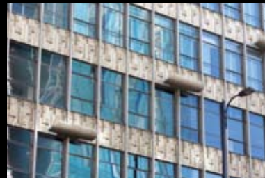
SBQ Exterior detail
