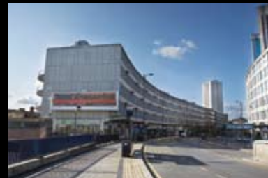
SBQ view from New Street Station
